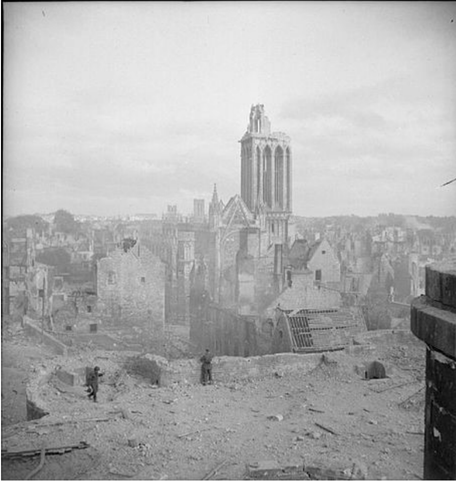
A general view of Caen showing the extensive damage caused by Allied bombing, 9 July 1944. By No 5 Army Film and Photographic Unit, Stewart (Maj) [Public domain], via Wikimedia Commons
